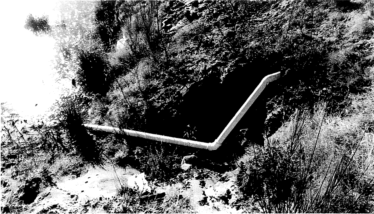
Figure 1. Drainage pipe in northern end of CWM site.
