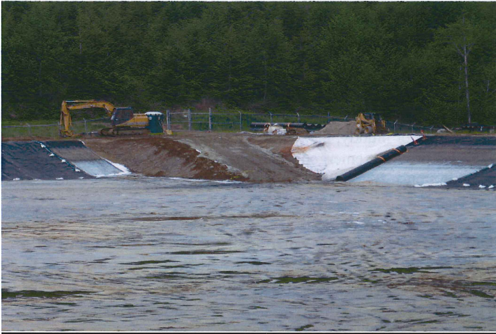
Installing new Hypalon liner in Raw Water Reservoir
