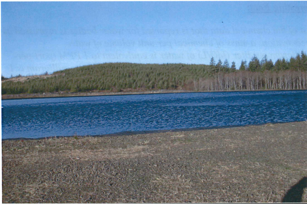
16 Million Gallon Raw Water Reservoir
