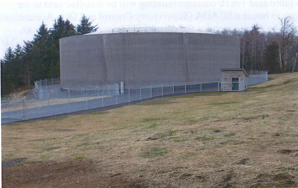
3.5 Million Gallon South Water Reservoir
