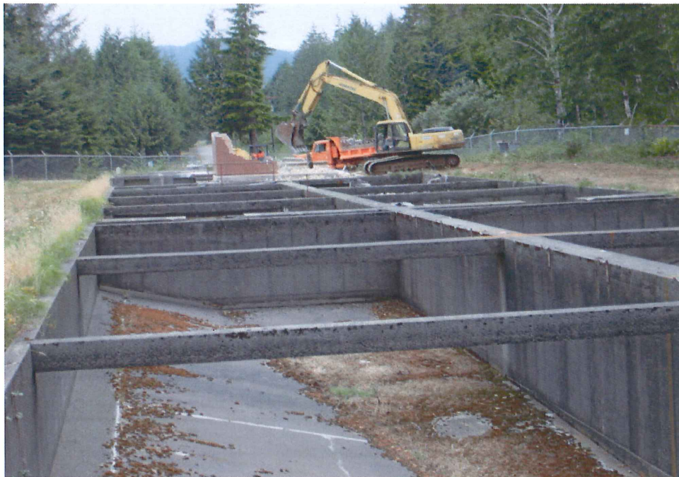
Old settling ponds during the demo process
