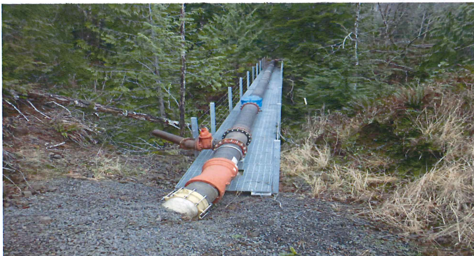
Big South Fork 16" Ductile Pipeline Crossing
