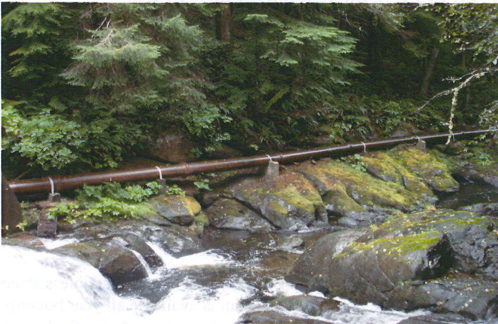
24inch DI pipe after realignment below L&C Dam
