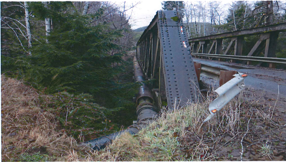
Bridge 7 with L&C Pipeline Crossing
