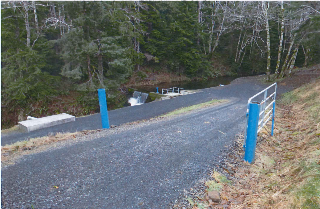
Little South Fork Dam
