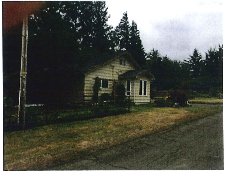
SE Jetty Residence Looking South
