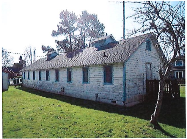
View of subject facing southwest
