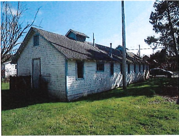
View of subject facing southeast
