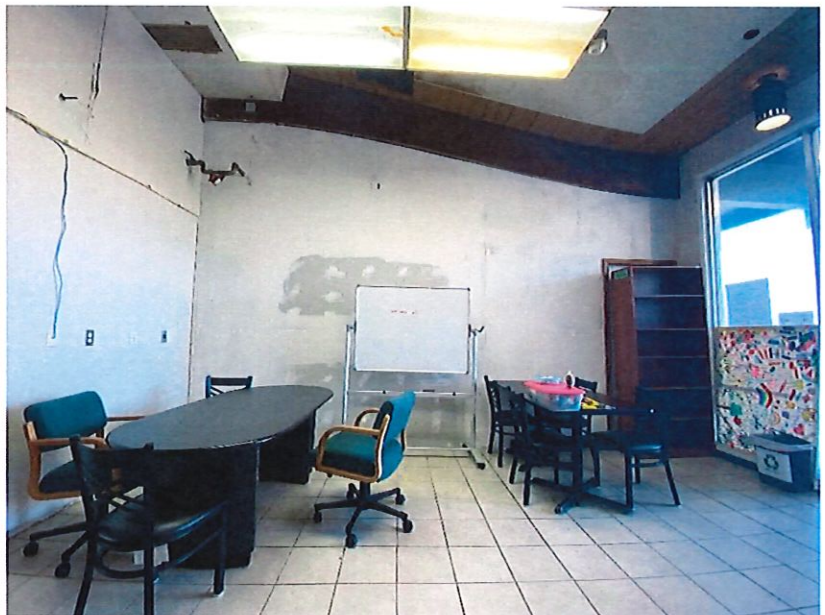
Image 2: Library backroom as of 9/7/22 waiting for finishing touches and paint.
