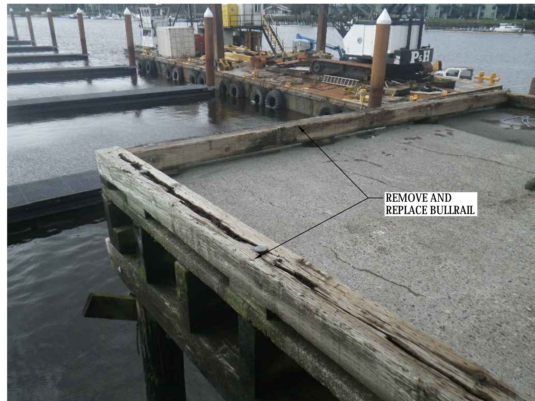
4 PHOTO - WEST TRESTLE BULLRAIL S-06 SCALE: NTS
