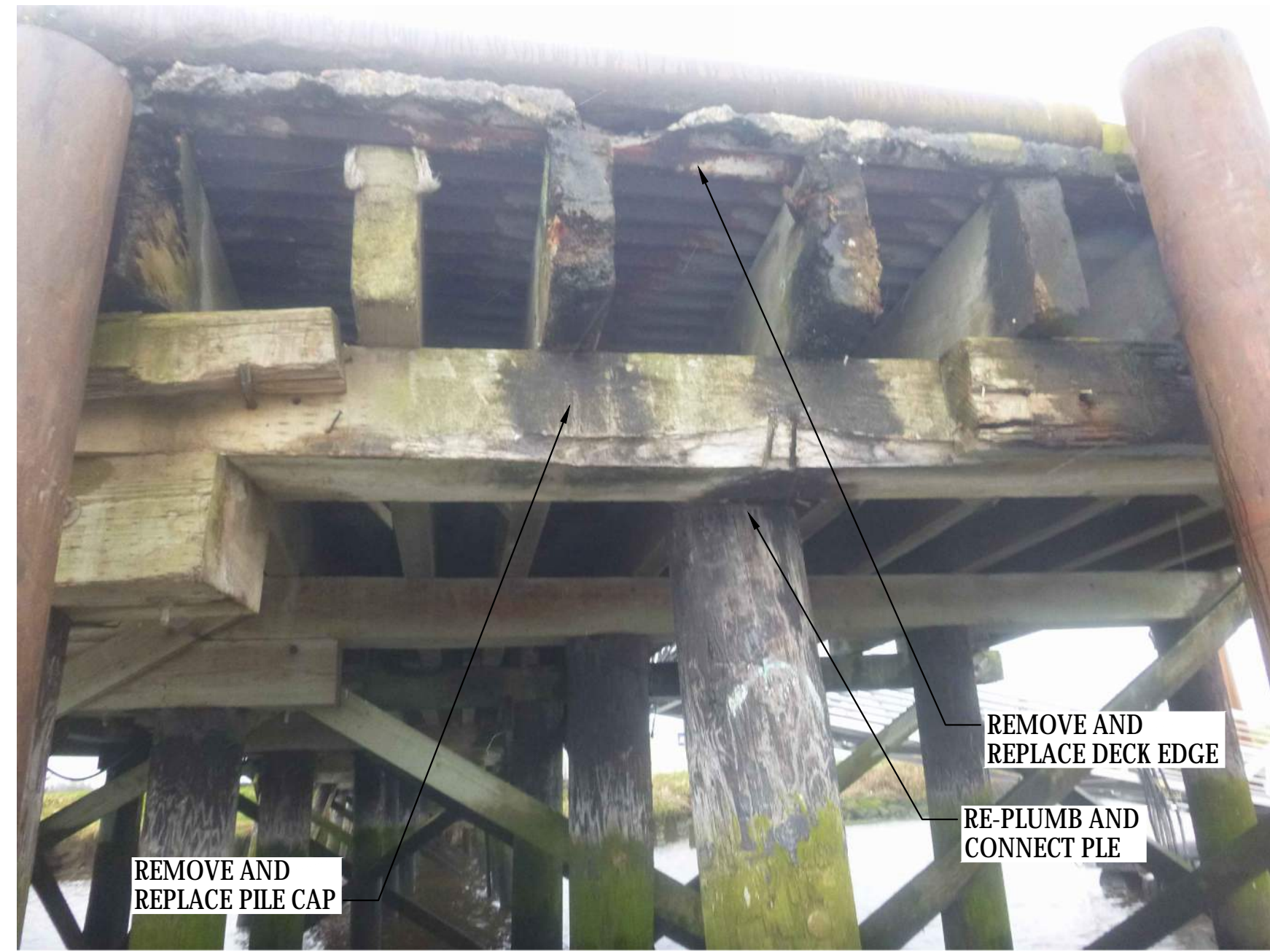
7 PHOTO - NORTH EDGE OF WEST TRESTLE S-06 SCALE: NTS
