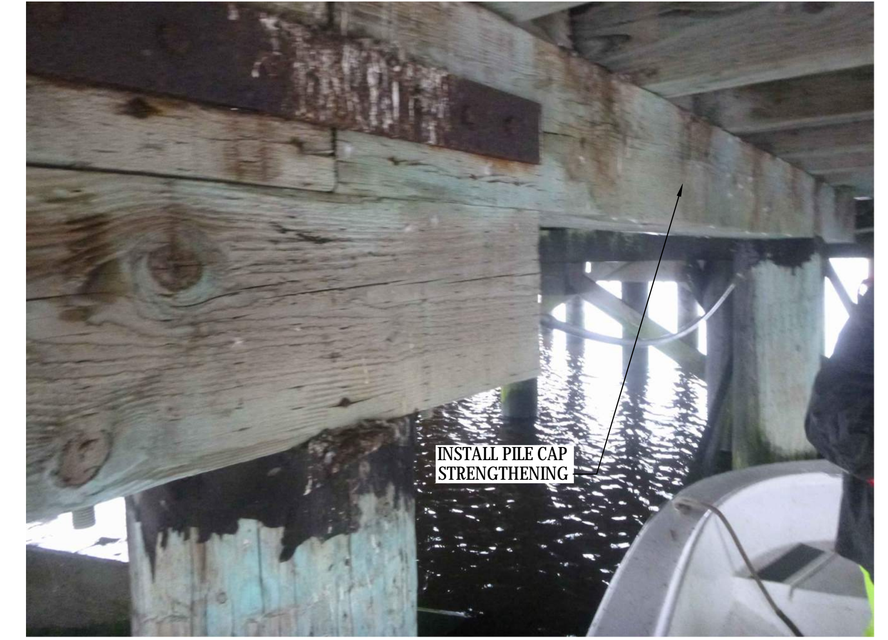
3 PHOTO - WORK PIER PILE CAP WP1 S-06 SCALE: NTS
