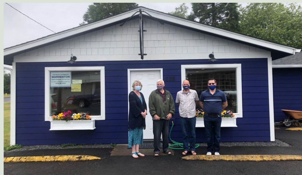
Above: a building renovation in downtown Warrenton, funded in part by funds from the WURA. Source: City of Warrenton
