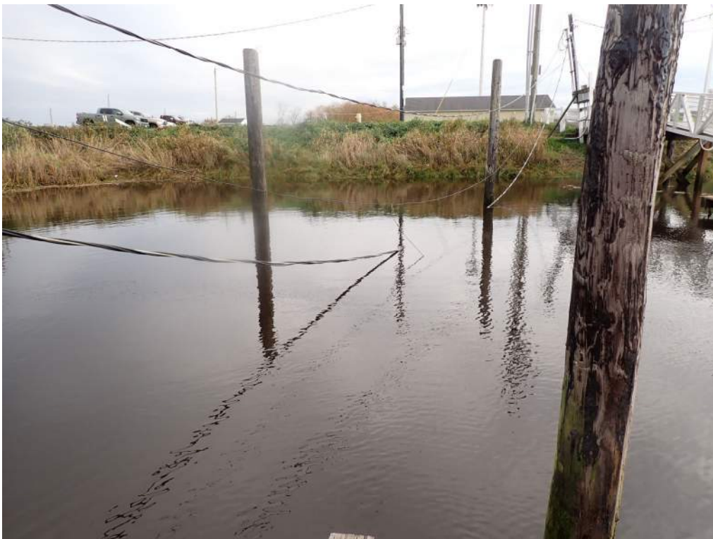
Photograph 32– Submerged Utility Line Near Northwest Marina Entrance
