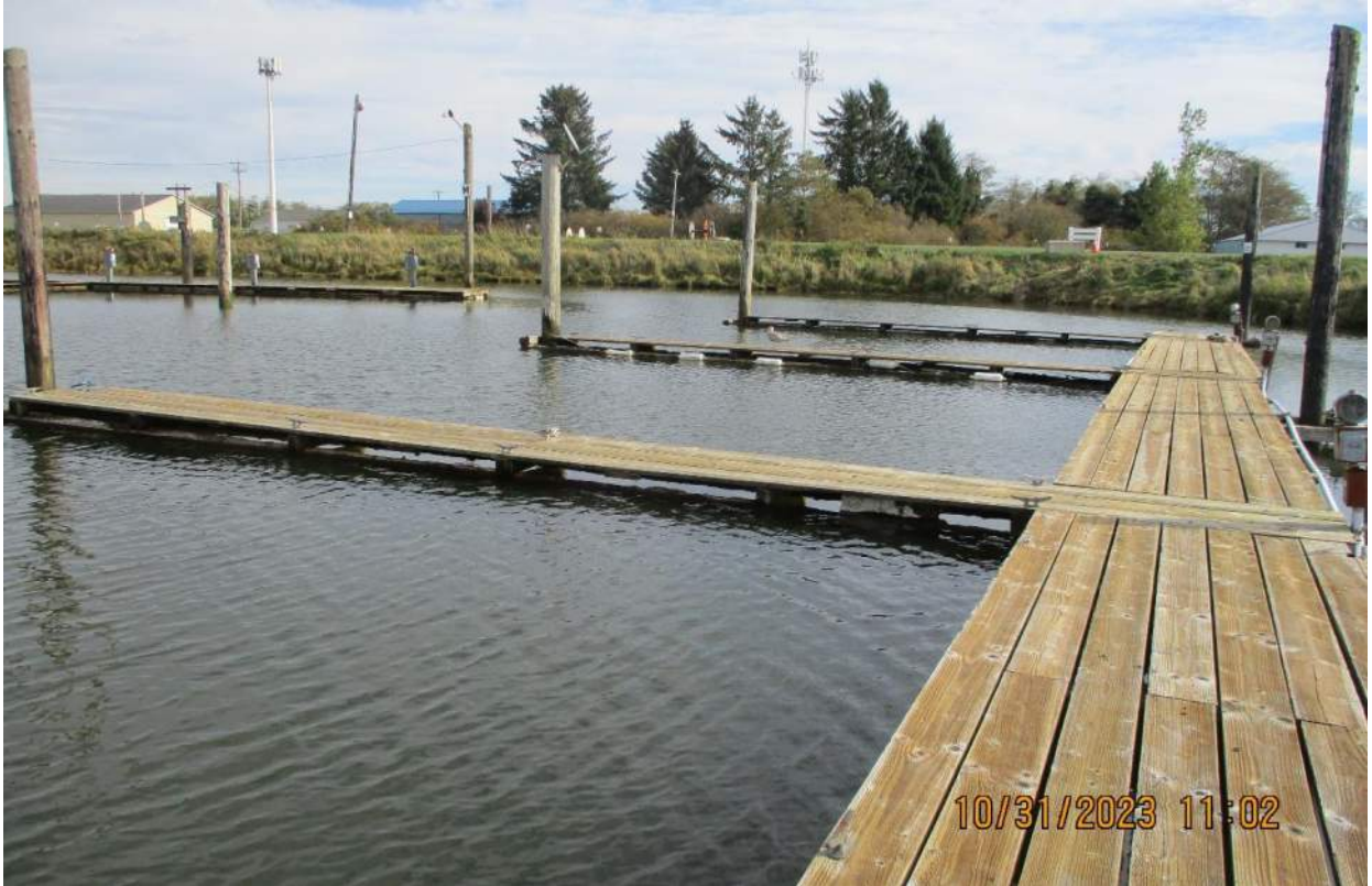
Photo 13: Another example of finger pier decking continuous into the walkway.
