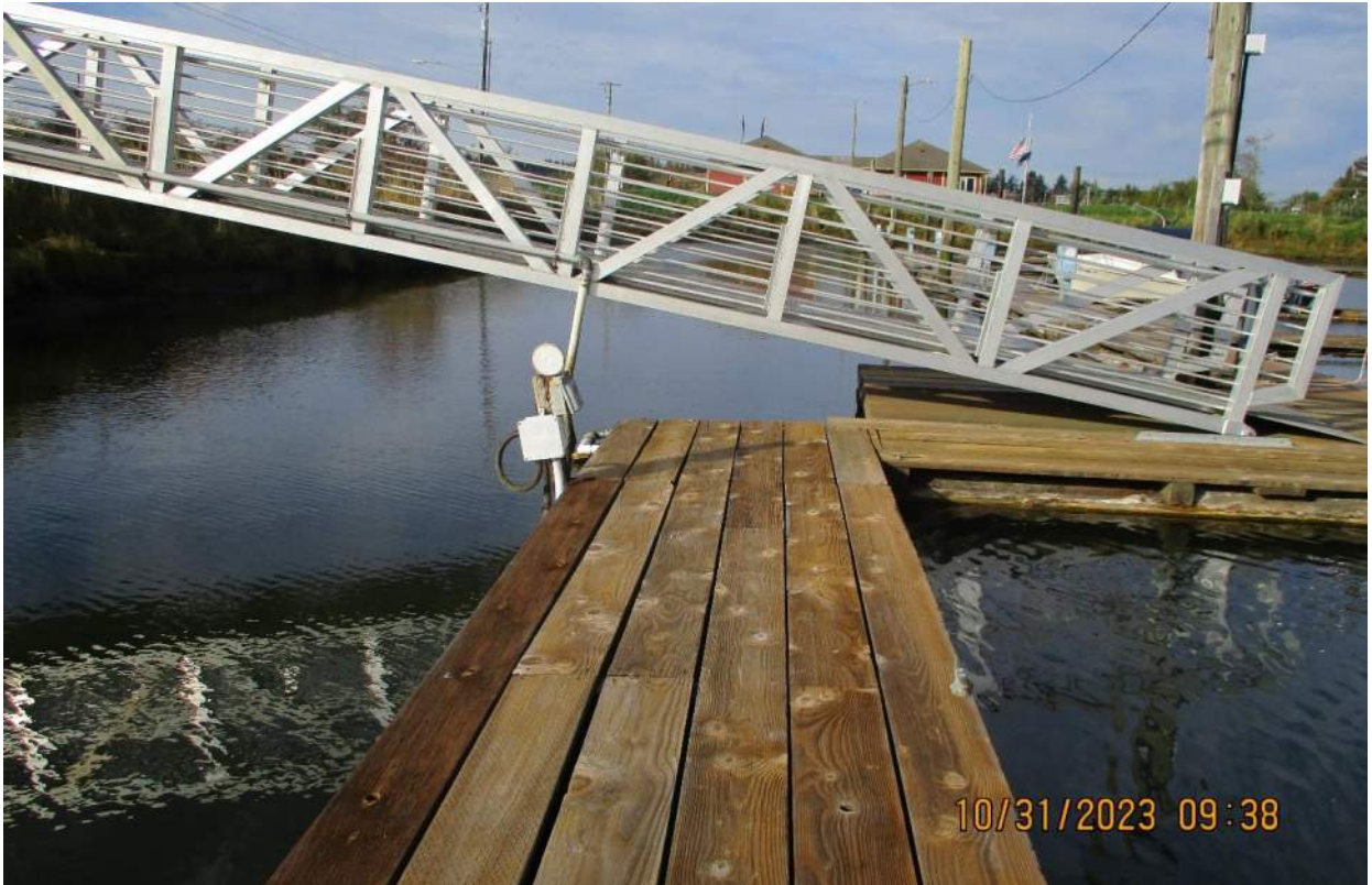
Photo 18: Typical condition of the gangway
