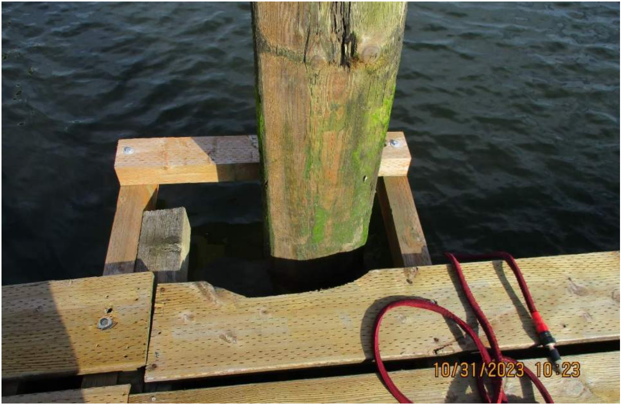
Photo 3: Recently replaced wooden pile hoop.
