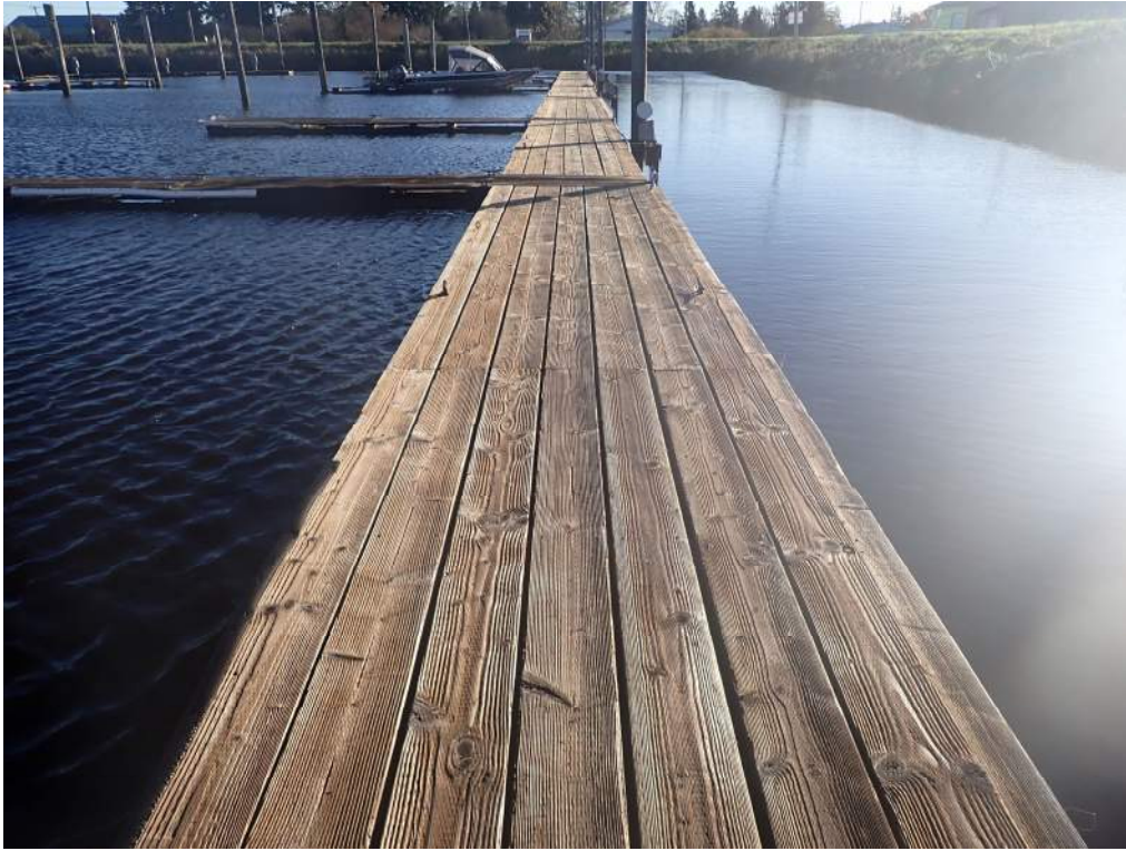
Photograph 7– Typical Main Floating Dock Condition
