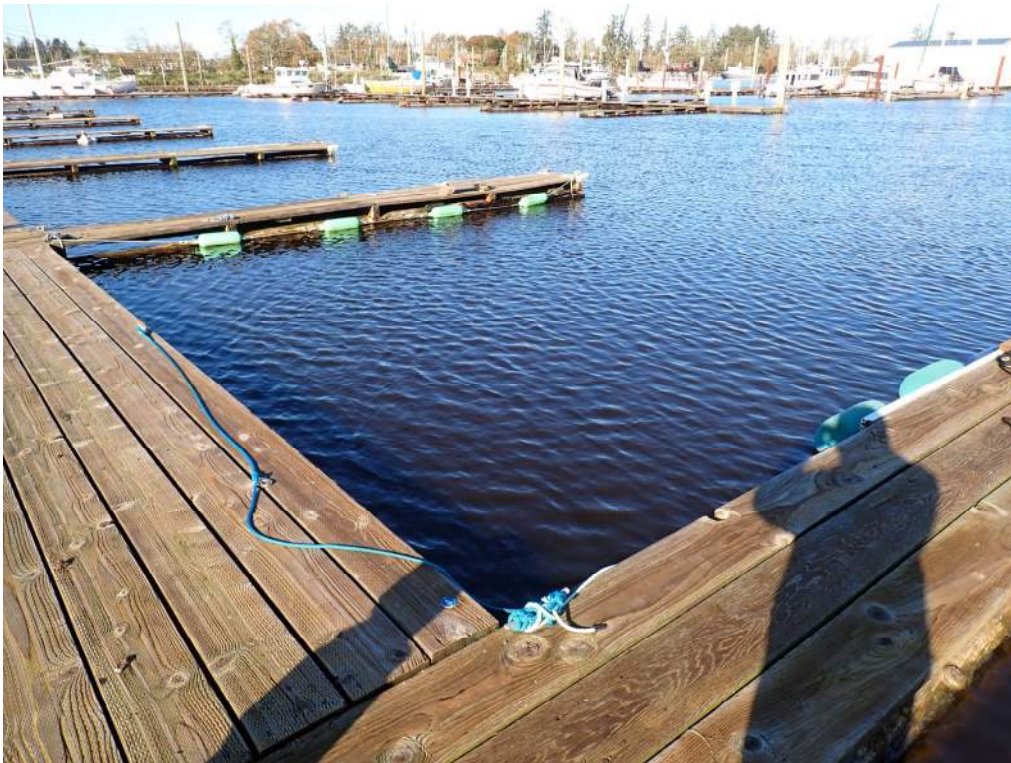
Photograph 8– Typical Finger Pier Condition
