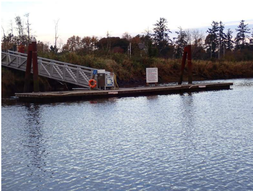
Photograph 6– Pump Out Dock, Looking Northwest
