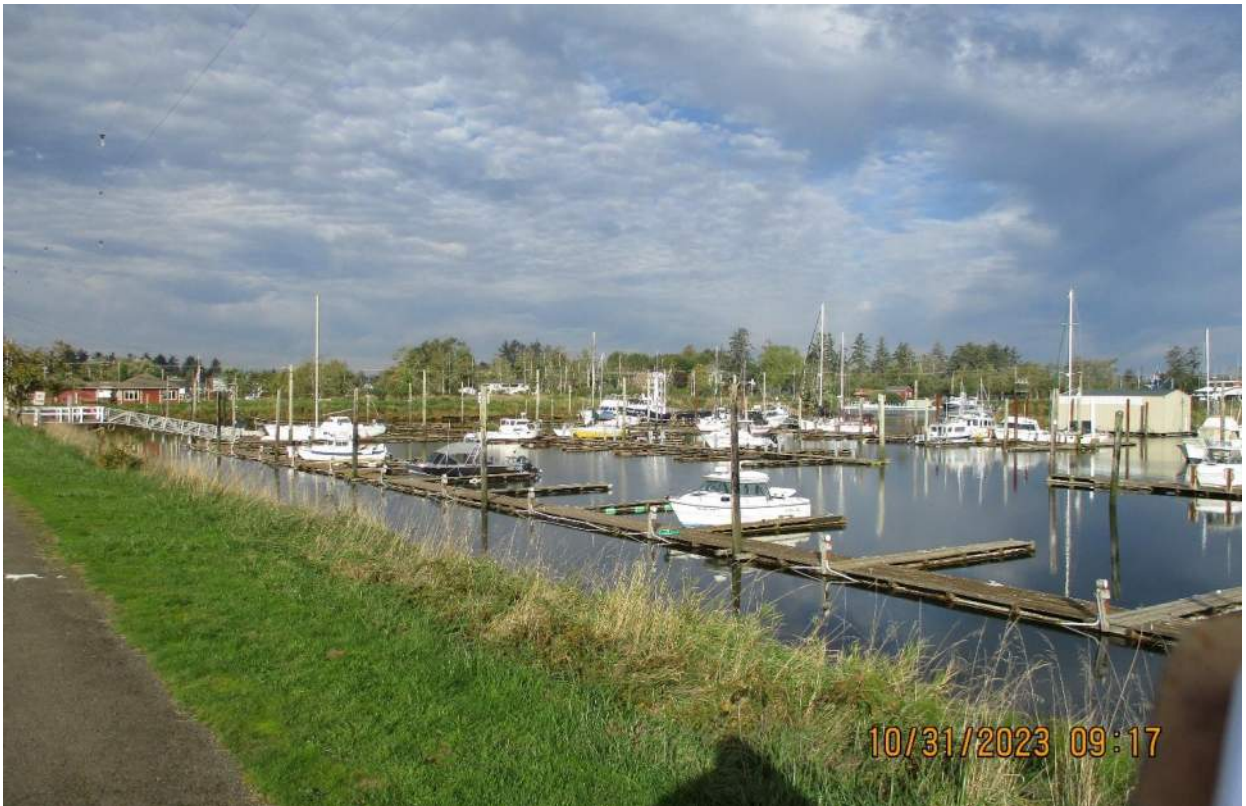
Photo 20: Overall view of the marina. Note the PVC conduits in the water.
