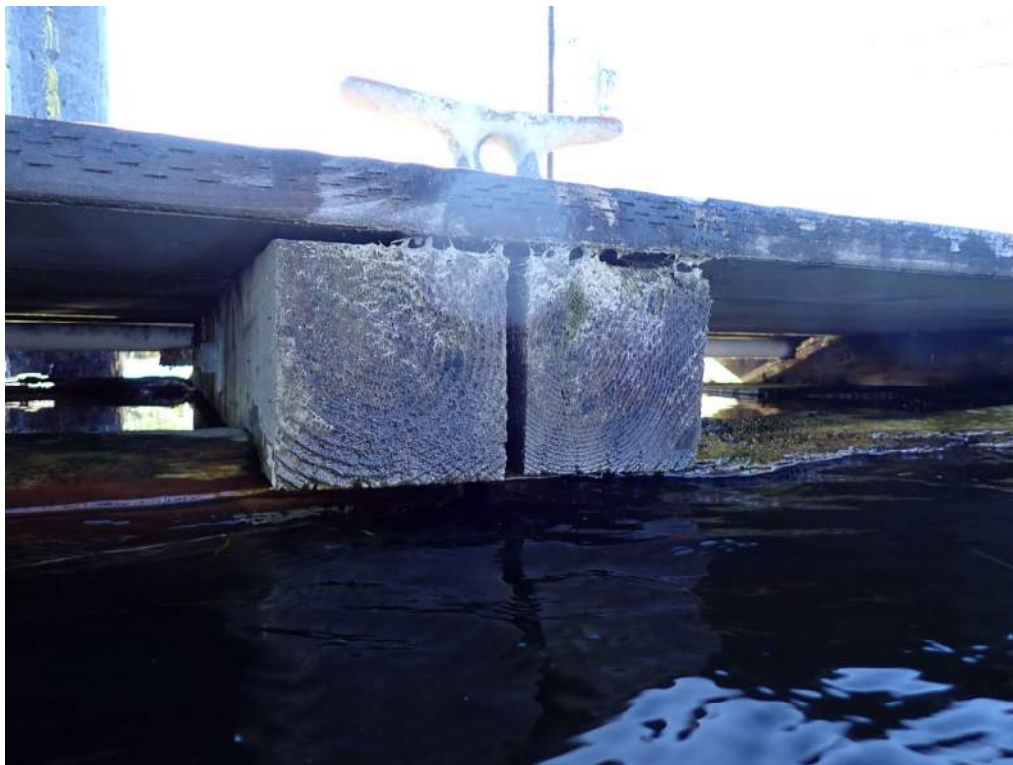
Photograph 16– Typical Transverse Timber Support
