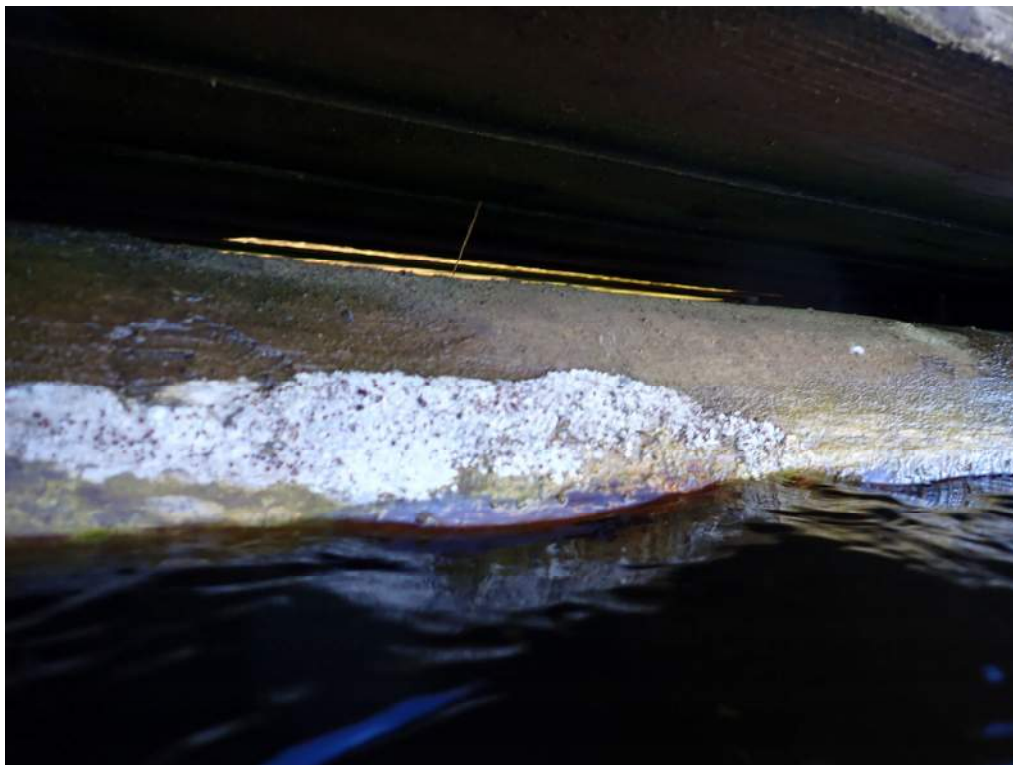
Photograph 14– Typical Timber Float at Waterline
