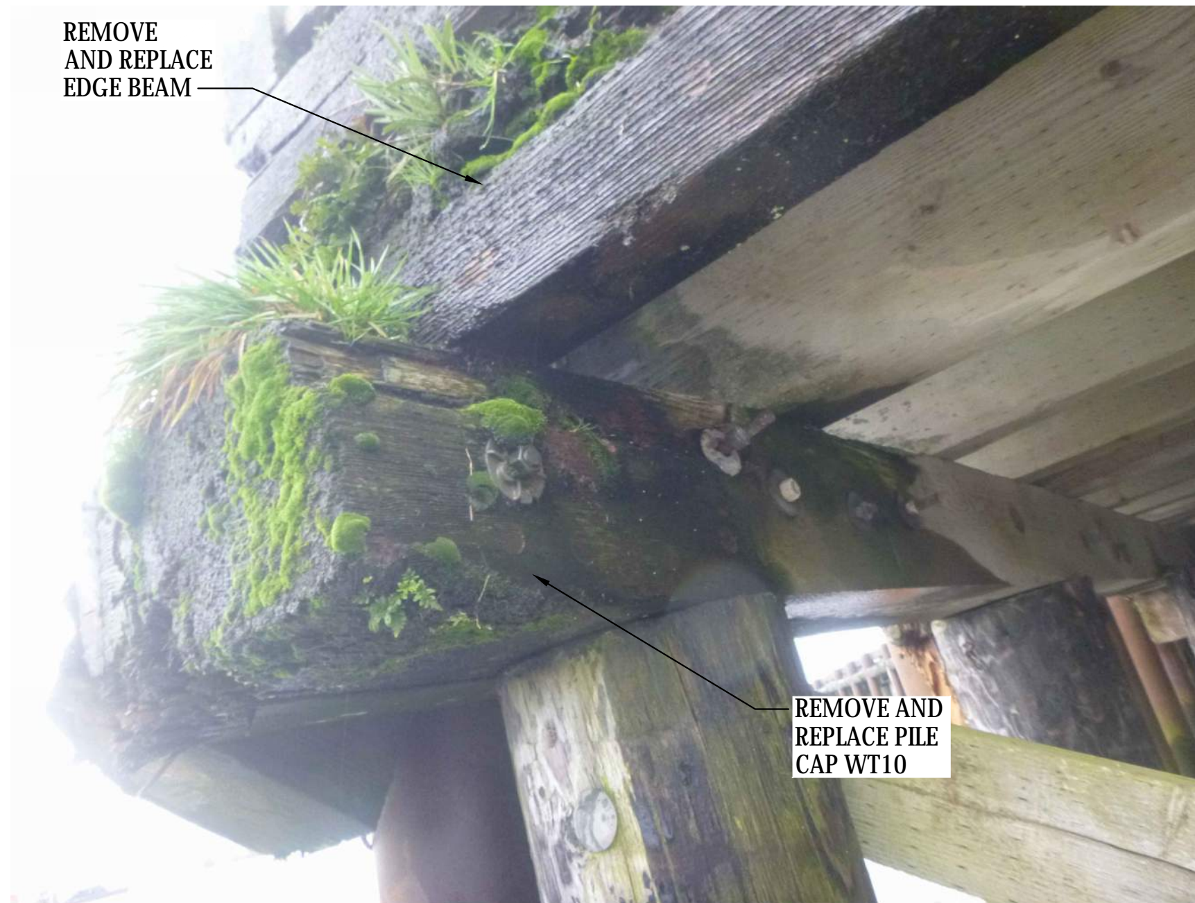
5 PHOTO - WEST TRESTLE PILE CAP WT10 S-06 SCALE: NTS
