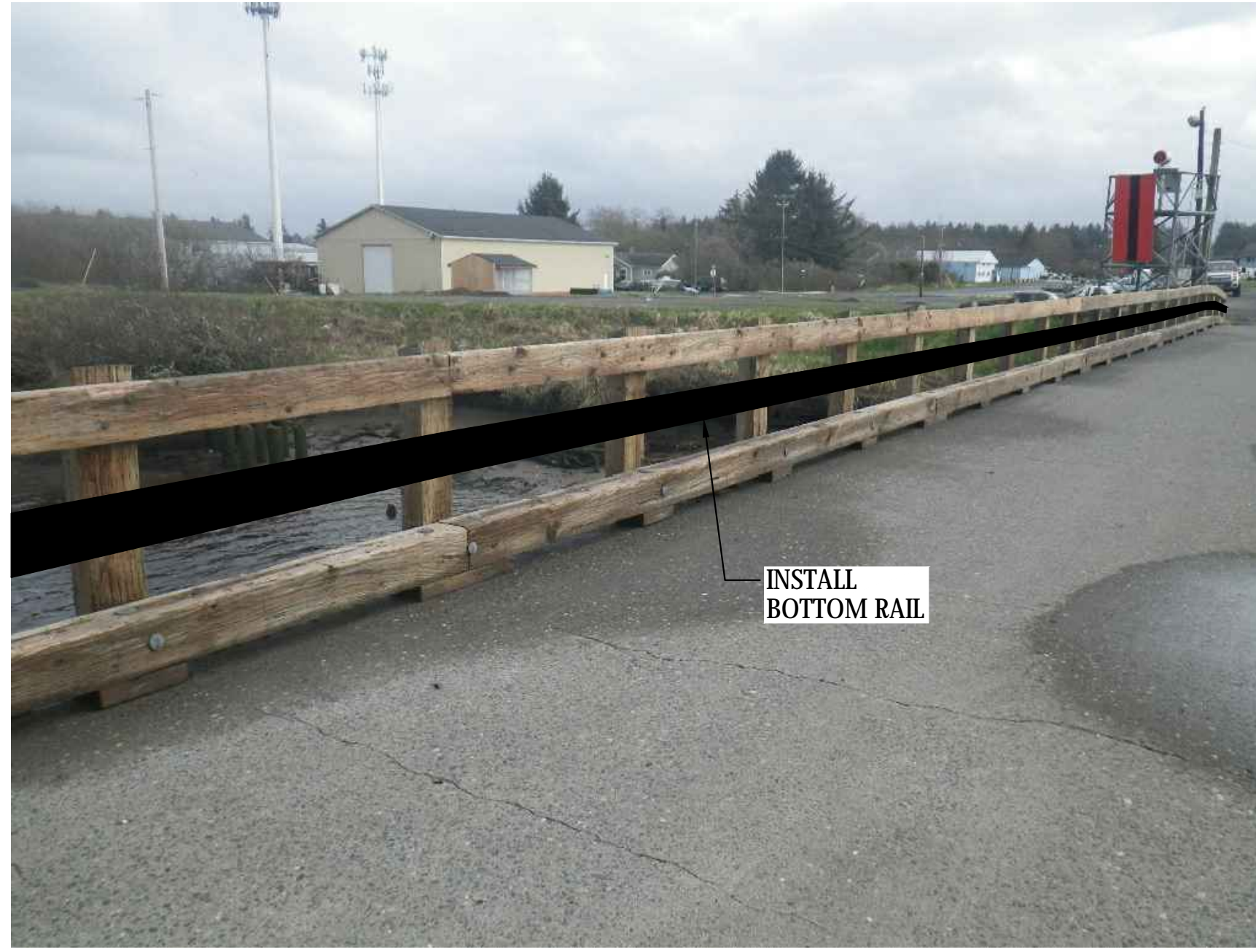
2 PHOTO - WEST TRESTLE RAILING S-05 SCALE: NTS
