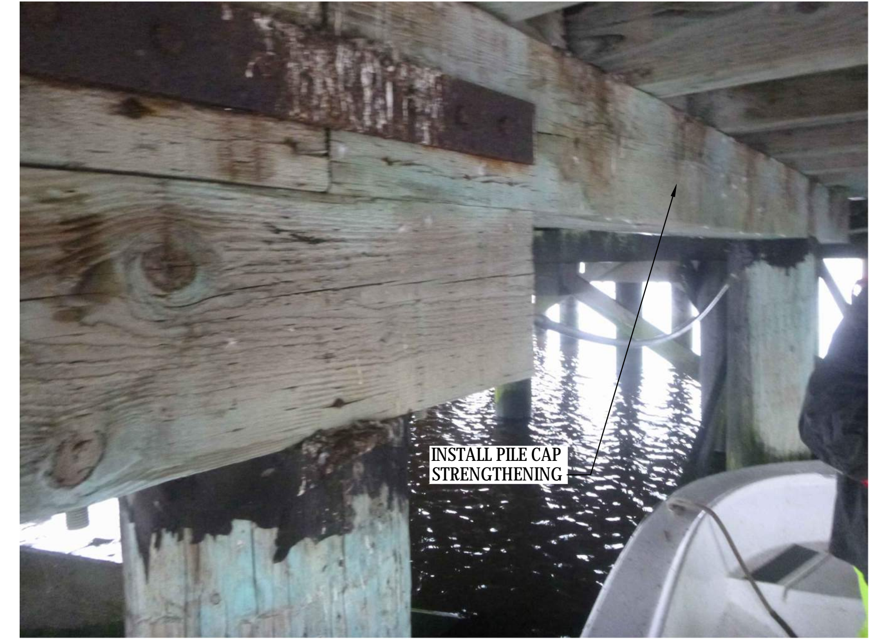
3 PHOTO - WORK PIER PILE CAP WP1 S-06 SCALE: NTS
