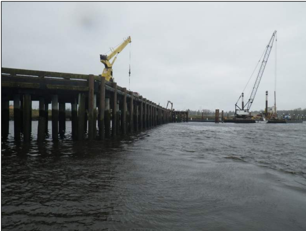
Photo 4. Work Pier (River Side) Looking West
