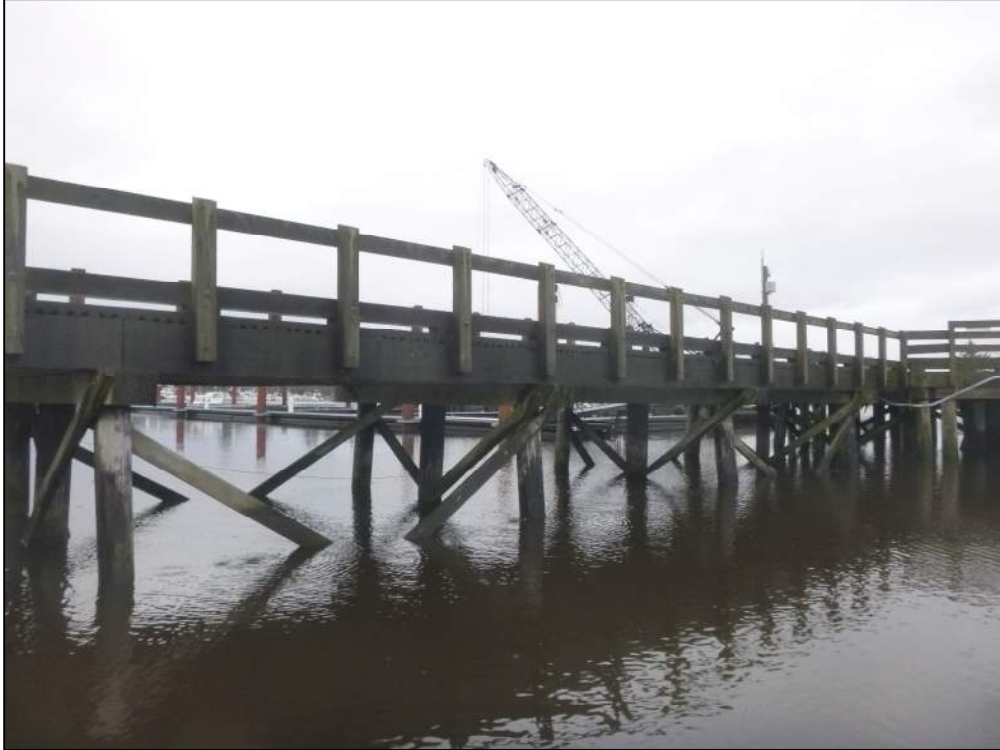
Photo 1. West Trestle Looking Northwest
