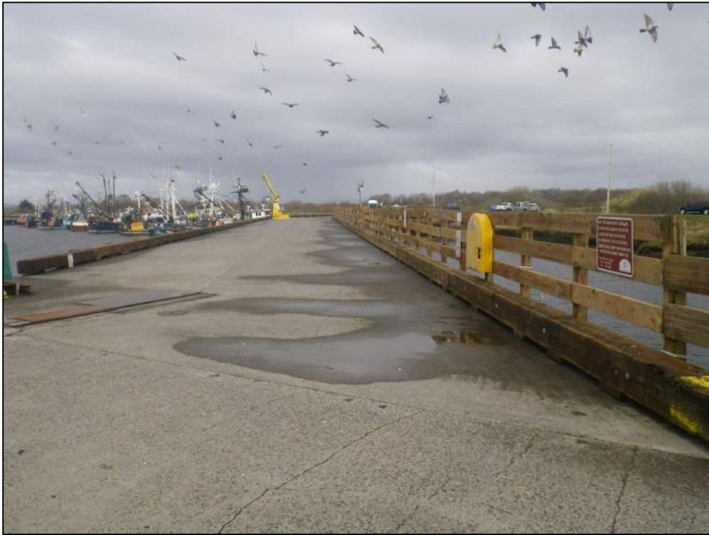
Photo 37. Work Pier Typical Railing And Bullrail
