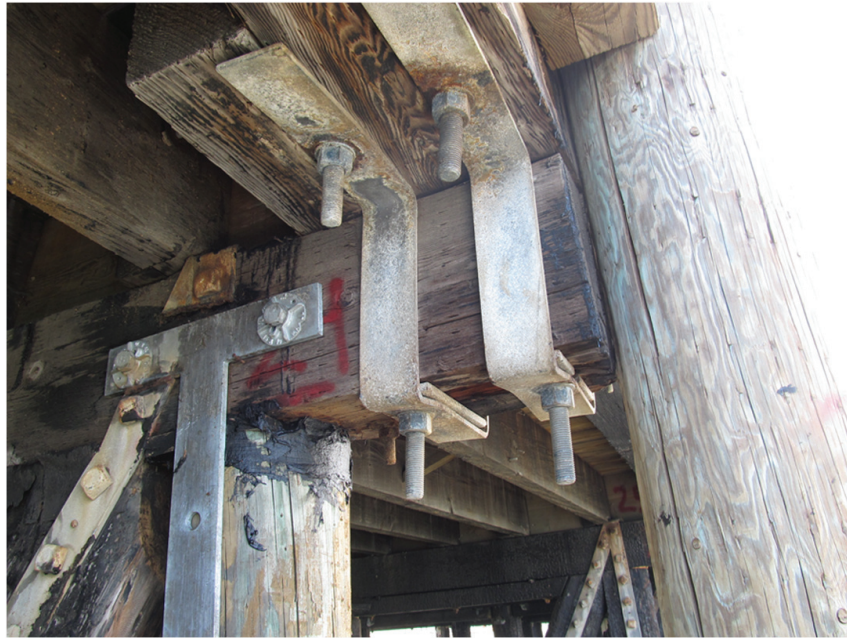
Fig. A-3. Typical connection detail of a timber wharf showing steel elements connecting a plumb fender and a battered pile to a pile cap (left); steel strapping securing a mooring cleat to the pile cap is also shown on the right Source: Courtesy of Simpson Gumpertz & Heger, Inc., reproduced with permission.
