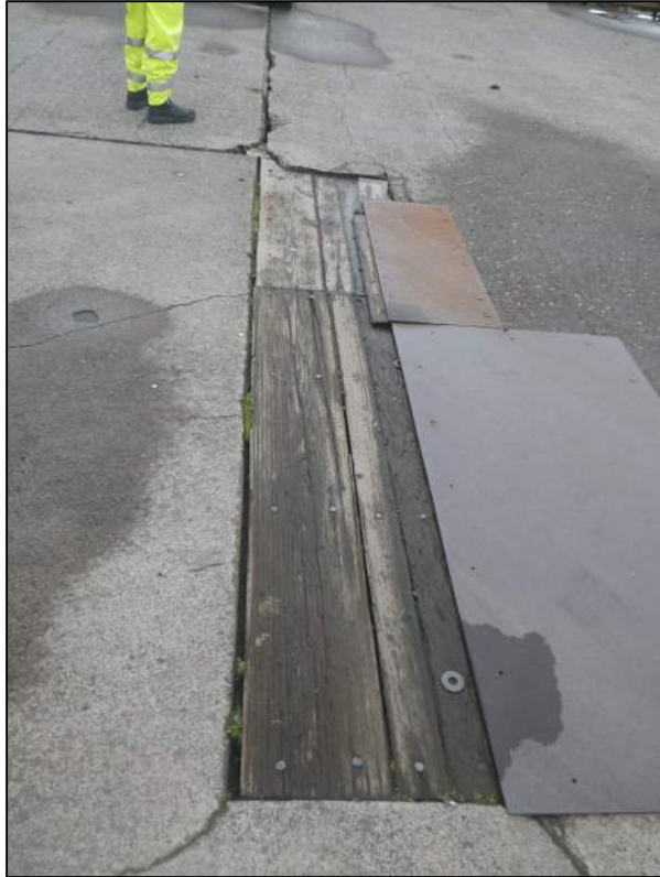
Photo 27. West Trestle Removed Deck At WT8
