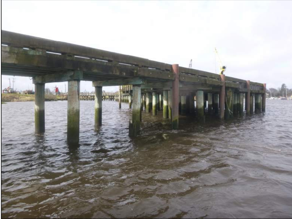
Photo 5. East Trestle Looking West
