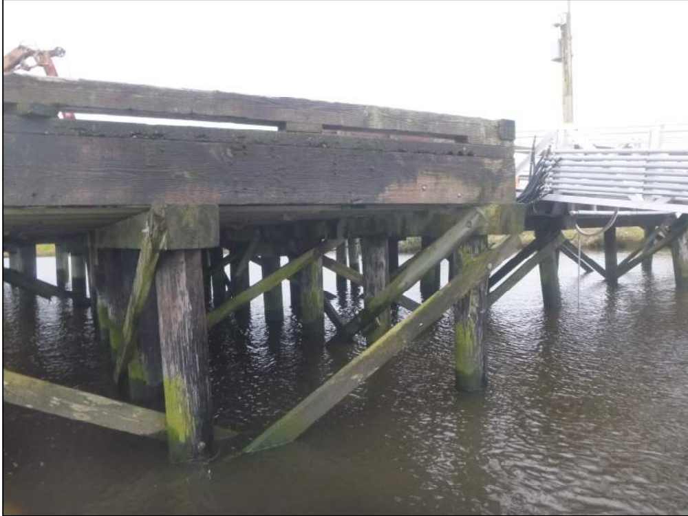
Photo 17. West Trestle Typical Bracing
