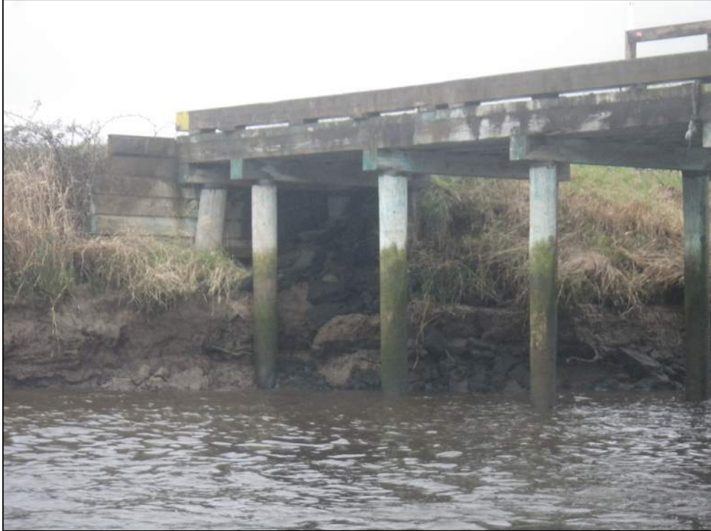
Photo 9. East Trestle Abutment
