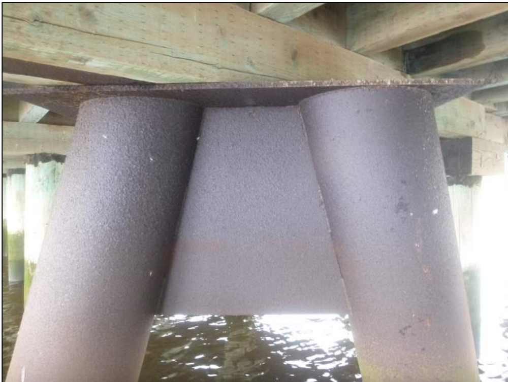
Photo 18. Typical Steel Battered Pile Pair (Bent WP13)
