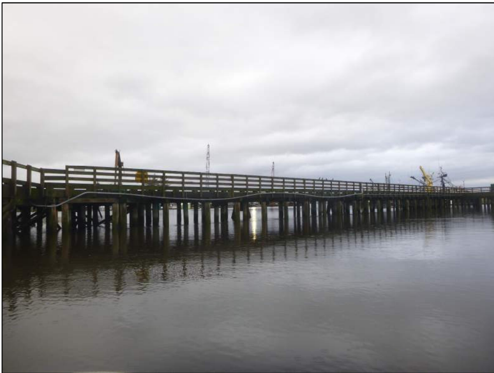
Photo 2. Work Pier Looking North
