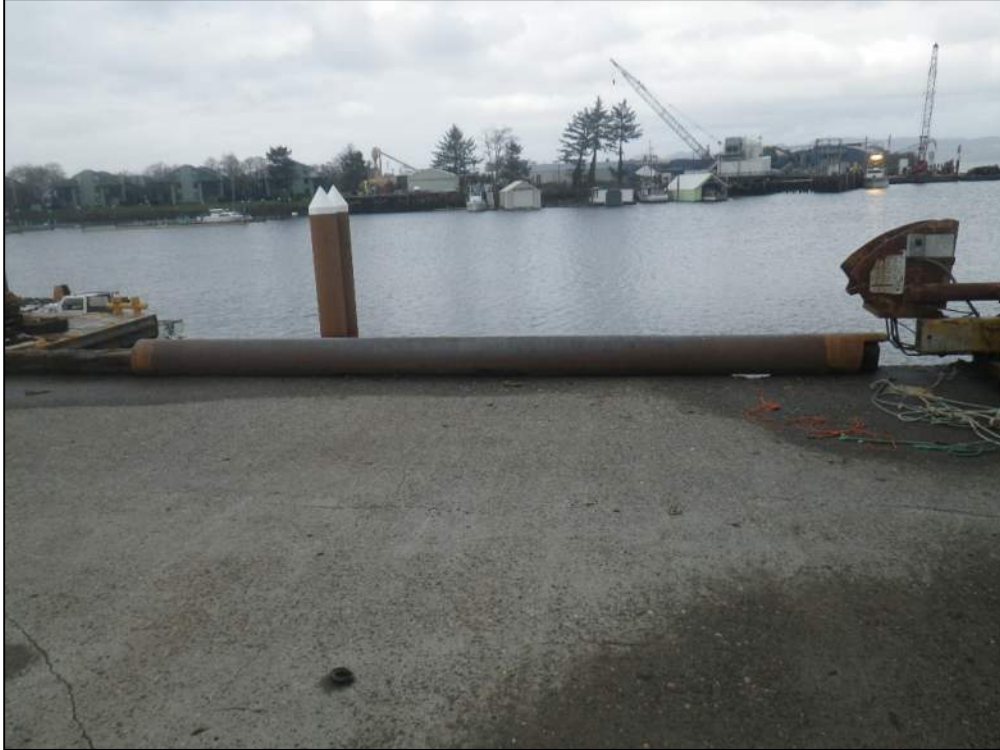
Photo 35. West Trestle Steel Bullrail At Bent WT10
