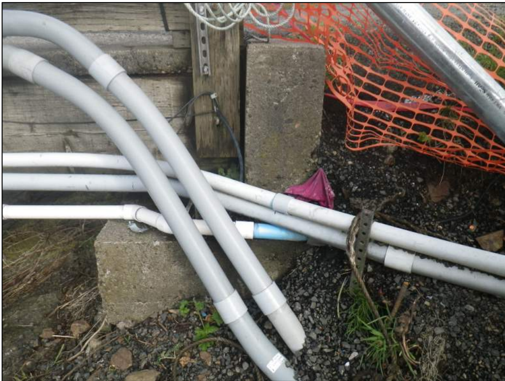
Photo 8. West Trestle Abutment Side View
