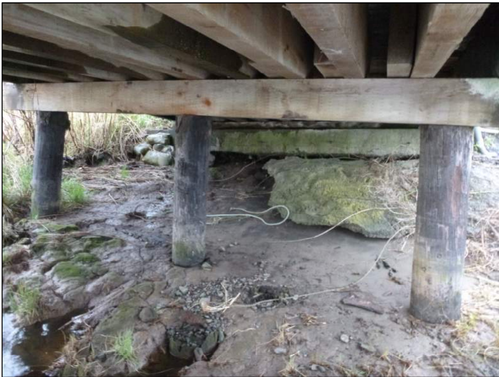
Photo 6. West Trestle Abutment
