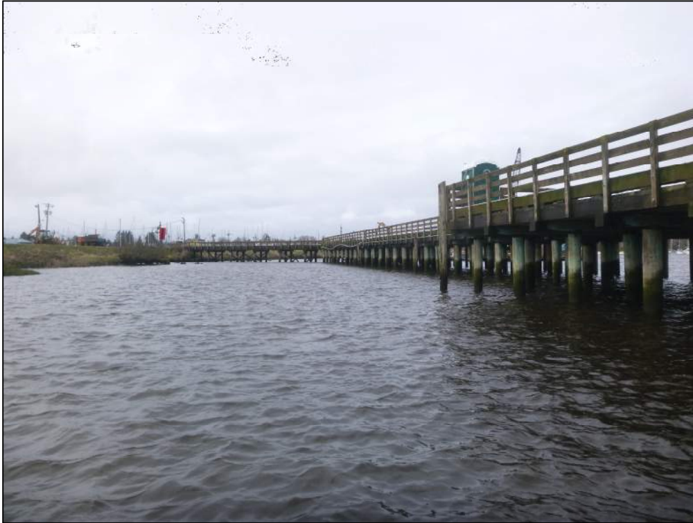
Photo 3. Work Pier (Shore Side) Looking West
