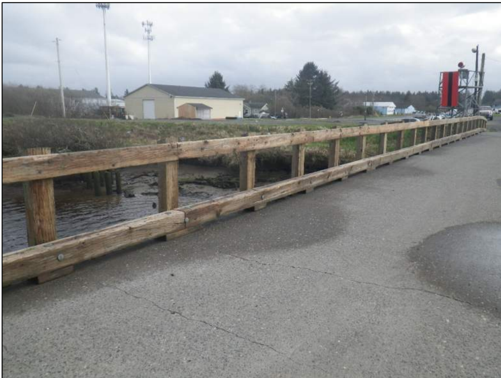
Photo 32. West Trestle Typical Railing And Bullrail
