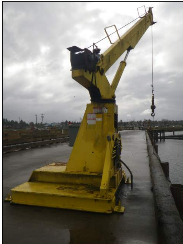
Photo 36. Work Pier Bullrail At River Side Edge
