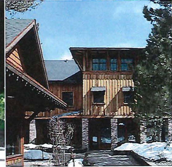
A modern interpretation of historic mining forms is appropriate for the Village Center.
