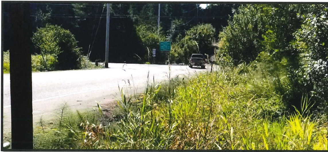
Figure 2: Sight Distance to the South at Marlin Avenue Access
