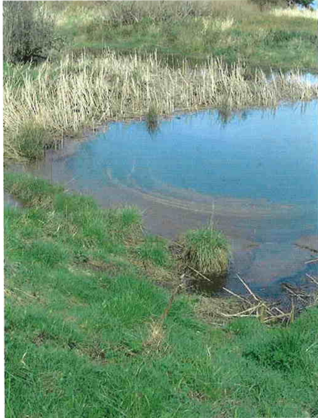
Tide Gate Under Water at High Tide at Alder Cove
