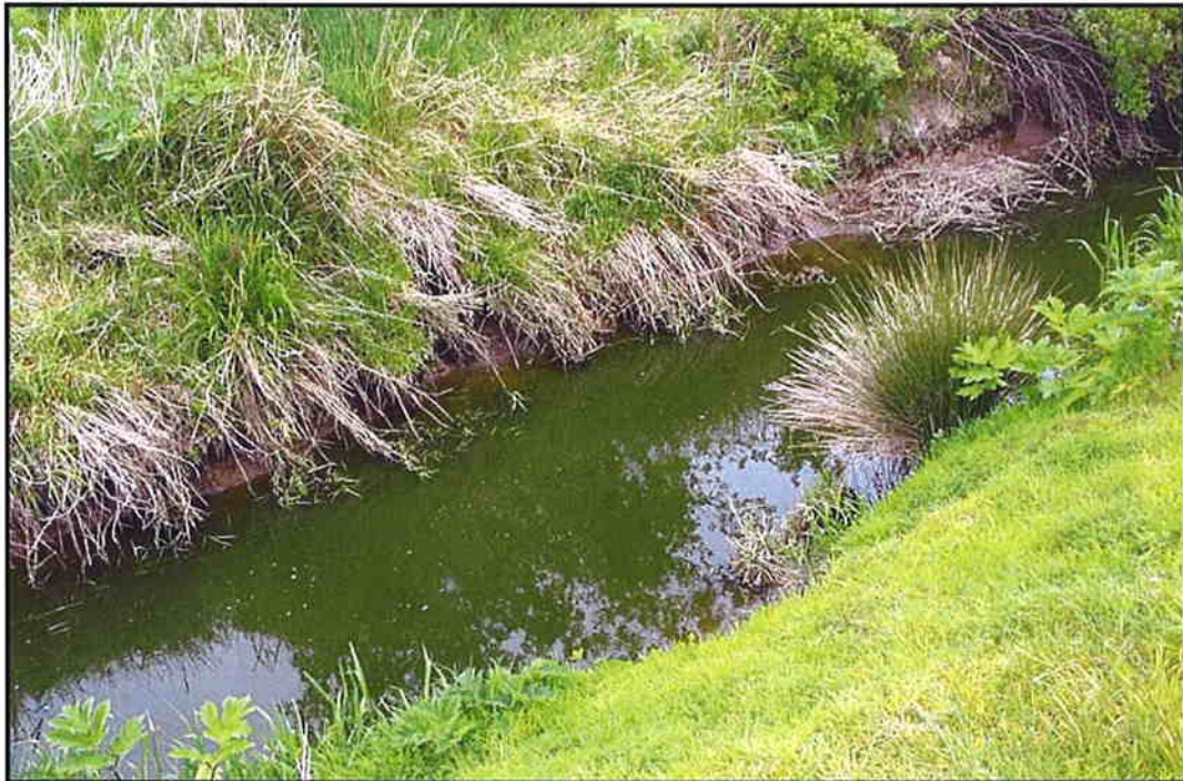
Figure 4: Constructed Effluent Channel
