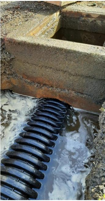
Public Works located a fire hydrant tie in on NE Skipanon Drive next to to a storage unit. The tie in was not previously marked on our GIS map.
