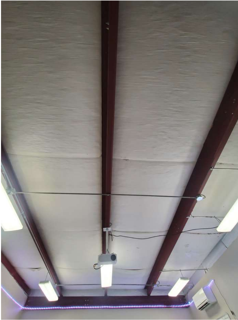
CEILING / ROOF ABOVE BREAK ROOM
