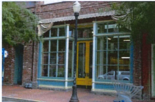
Historic storefront with painted wood windows and recessed entry (SW Oak St and 1st Ave)
