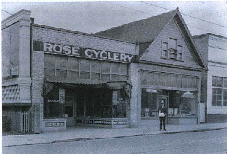
Historic photo from 1929 shows the benefits of retractable awnings and transom windows on a grey Oregon day.
