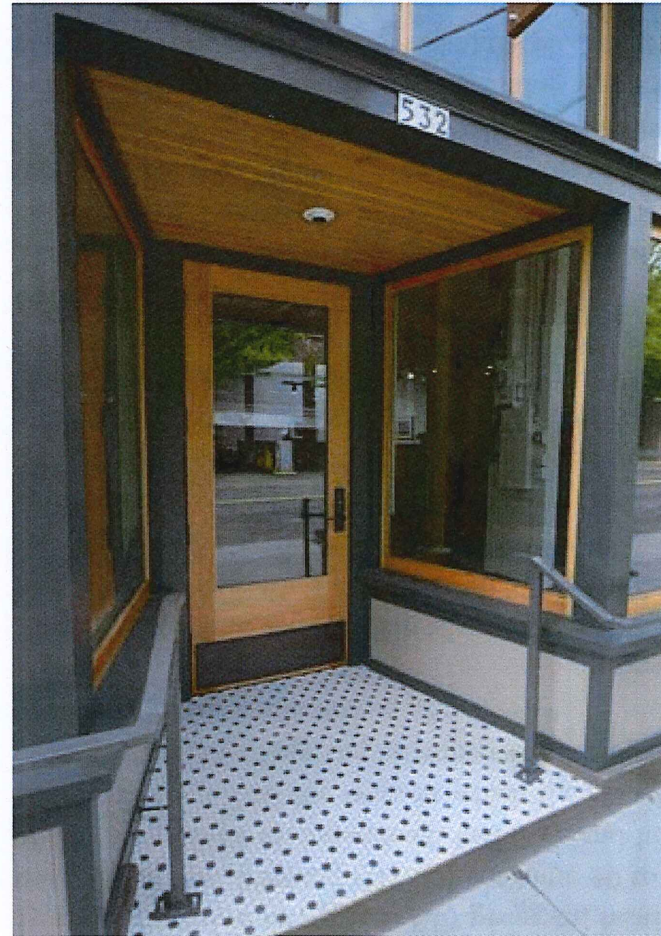
Storefront entry improvements built with local doug fir (SE Clay St and 6th Ave)
