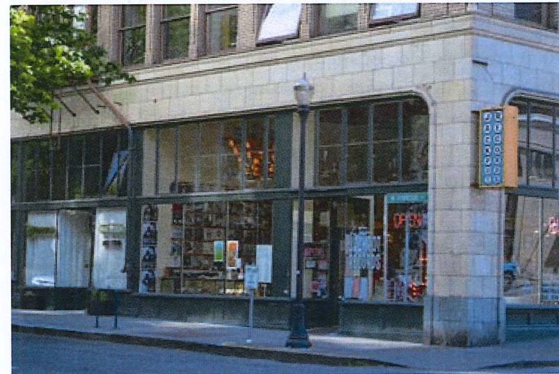
Elegant historic storefront with transoms above and wood window base gives a great sense of transparency to the interior. Note the operable transoms. (SW 9th Ave and Burnside St)
