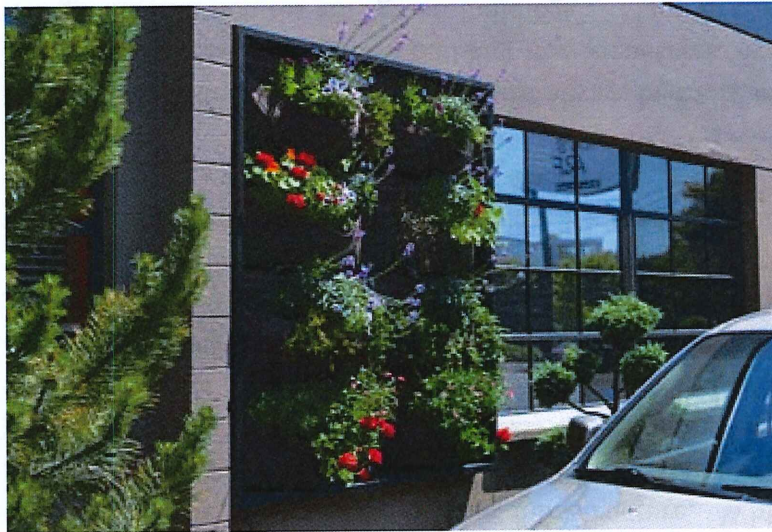
Vegetation wall at NW 18th Avenue and Pettygrove St
