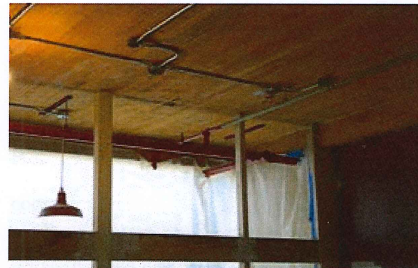
Exposing original wood ceilings add visual warmth. Relite windows to the ceiling allow natural light farther into interior spaces
