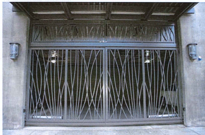
Parking Screen Wall
