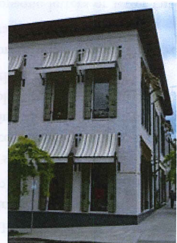
Retractable awnings are flexible especially for south and north facing glazing. (NW 23rd Ave and Flanders St)
