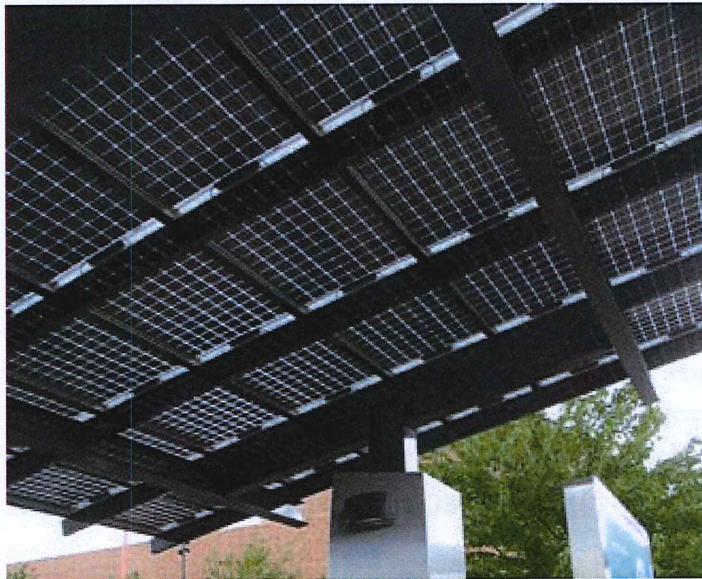
This solar array is used to charge electric cars (SE Water Ave)
