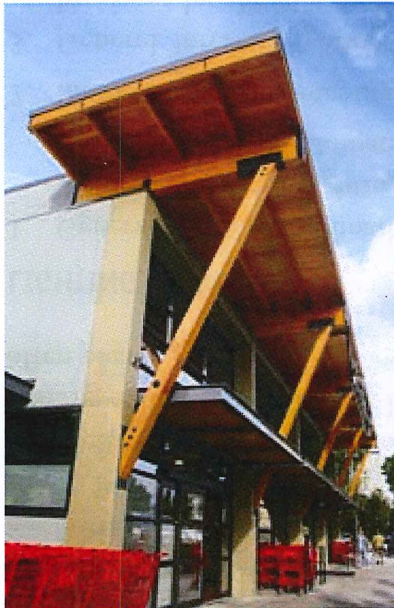
Double wooden south-facing canopies provide shade and weather protection for both windows and people. Photo by Stickleby Photo. (NE 41st and Halsey St)
