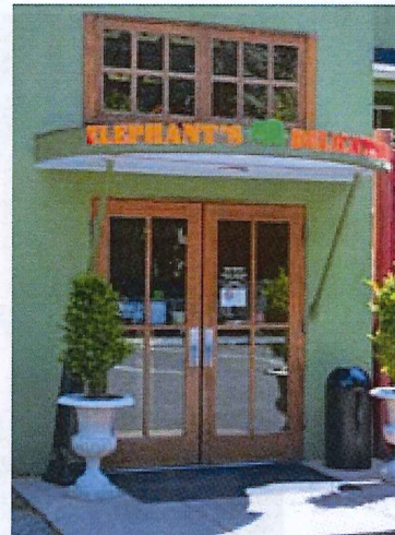
Exposed awning with signage (NW 22nd Ave and Davis St)
