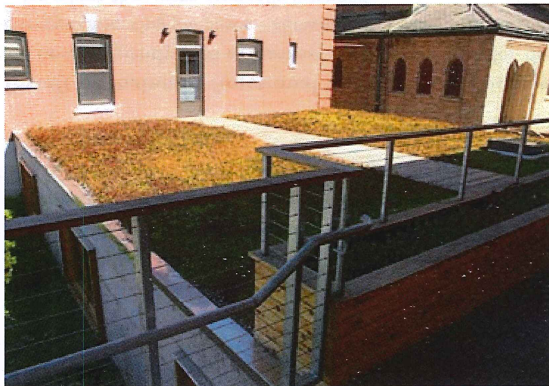
Deck and green roof (NE 8th Ave and Alberta St)
