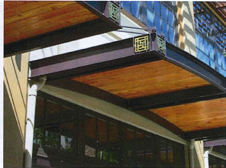
Remodeled storefront with clad windows and steel awning. Wood detail provides warmth to the underside. Photo by Rick Keating. (NW 12th Ave and Glisan St)
