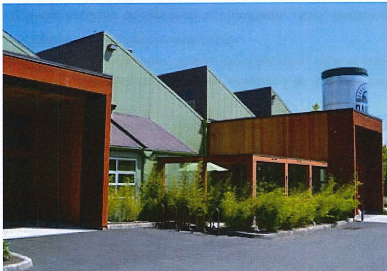
Unprotected mill finished steel and natural wood give warmth to this renovated industrial building. (NW 22nd Pl and York St)
