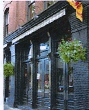
Retractable awnings give flexibility to weather and day lighting (SW 2nd Ave and Ash St)
