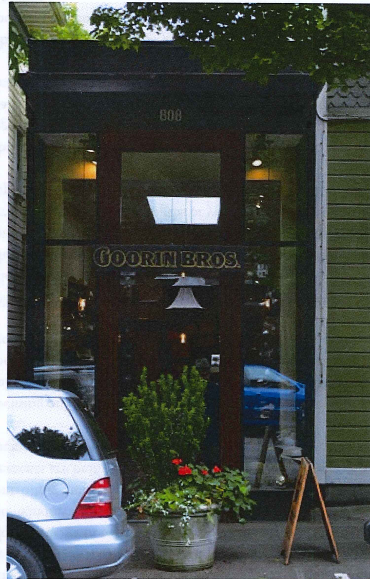
Narrow building maximizes day lighting with transom windows and a skylight (NW 23rd Ave and Johnson St)
