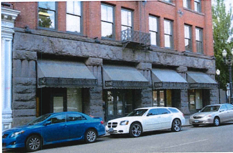
Awnings fit within storefront bays allowing the historic details of this building to be clearly visible (SW 2nd Ave and Ash St)
