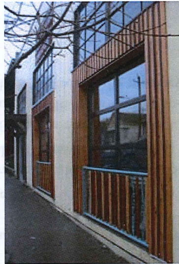
Infill areas of wood siding breaks up a long concrete facade while creating rhythm. (N Mississippi Ave)
