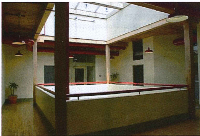
This atrium with skylights above allows light to travel deep into the building. (SW 1st Ave and Pine St)
