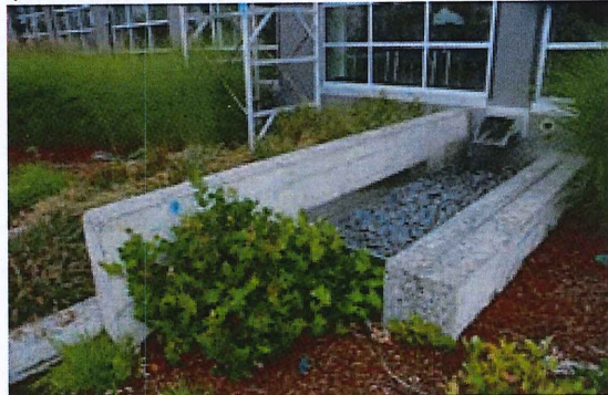
A roof drain integrates into the landscape as a flow-through planter. (SE Water Ave and Clay St)
