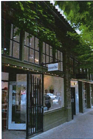
Storefront with nicely proportioned transom windows. (NW 23rd Ave and Johnson St)
