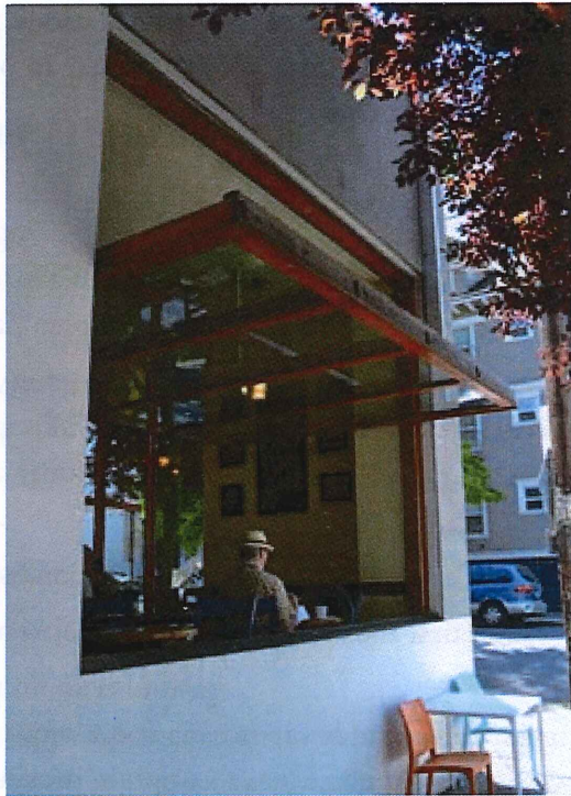
A display window cleverly converted to a large pivot window gives a sense of intimacy and protection like an awning. The window also energizes the street connection (NW Flanders St and 21st Ave)
