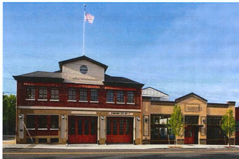
Carefully restored buildings along with new construction can work well to compliment each other. Changing brick color clearly defines these two buildings. (SE 11th Ave and SE Stark St)
