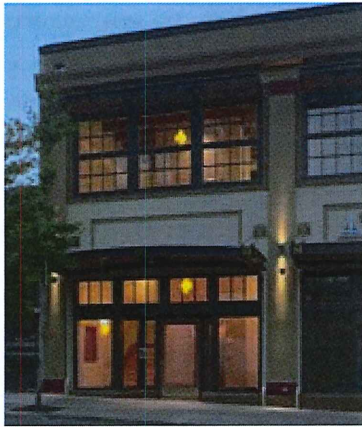
Up-down lighting located on the columns strengthens the rhythm of the Porter Building's bays. Photo by Rick Keating. (NW 12th Ave and Glisan St)
