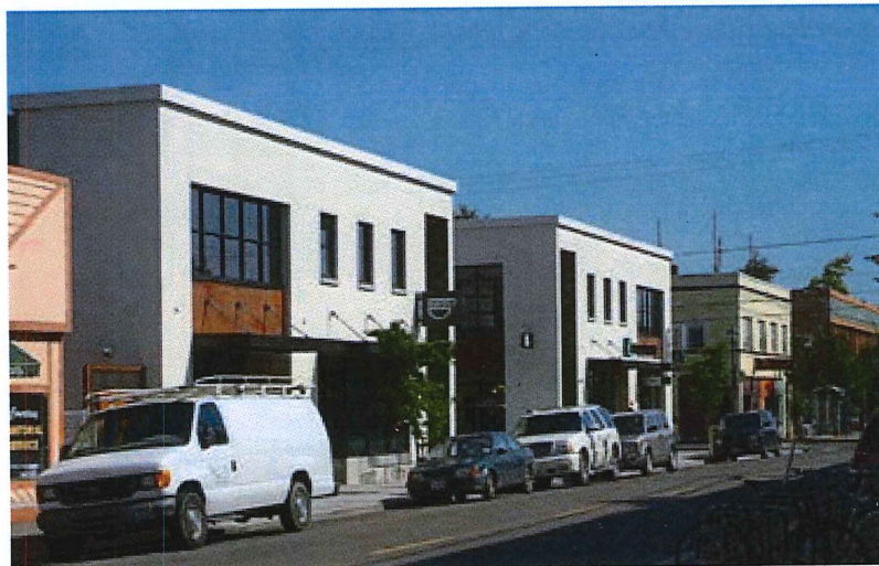
This infill project adopts the scale and massing of it's surrounding context (NE 18th Ave and Alberta St)
