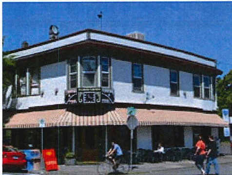
Fabric awning provides shading on south and west facades (NW 23rd Ave and Savier St)
