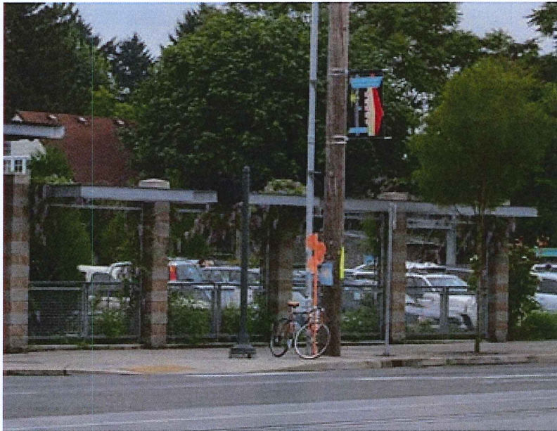
Screening can provide an attractive barrier between parking and sidewalks (N Interstate Ave and Rosa Parks Way)
