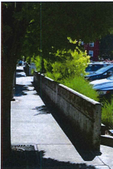
Parking Screen Wall
