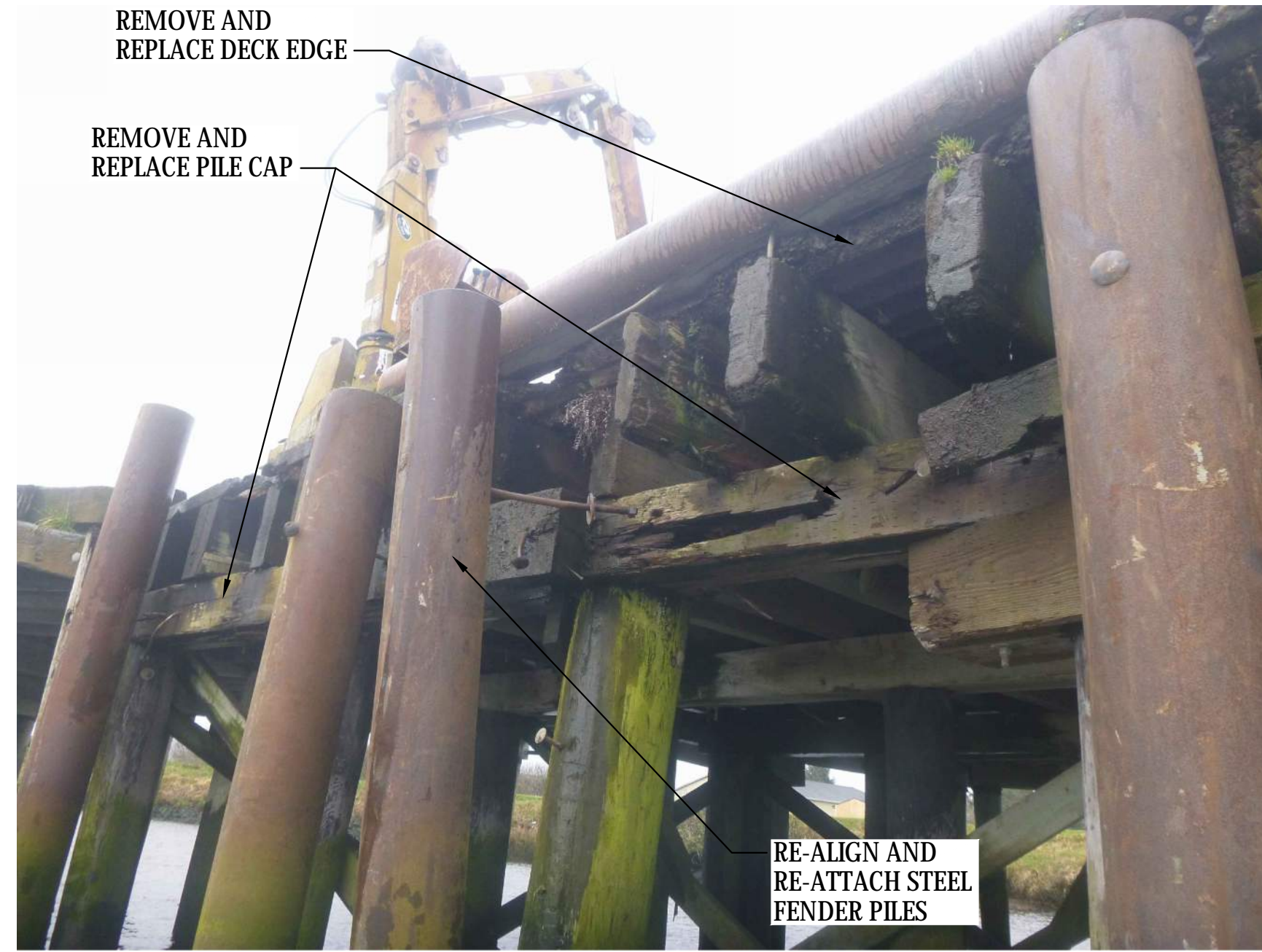
8 PHOTO - NORTH EDGE OF WEST TRESTLE S-06 SCALE: NTS
