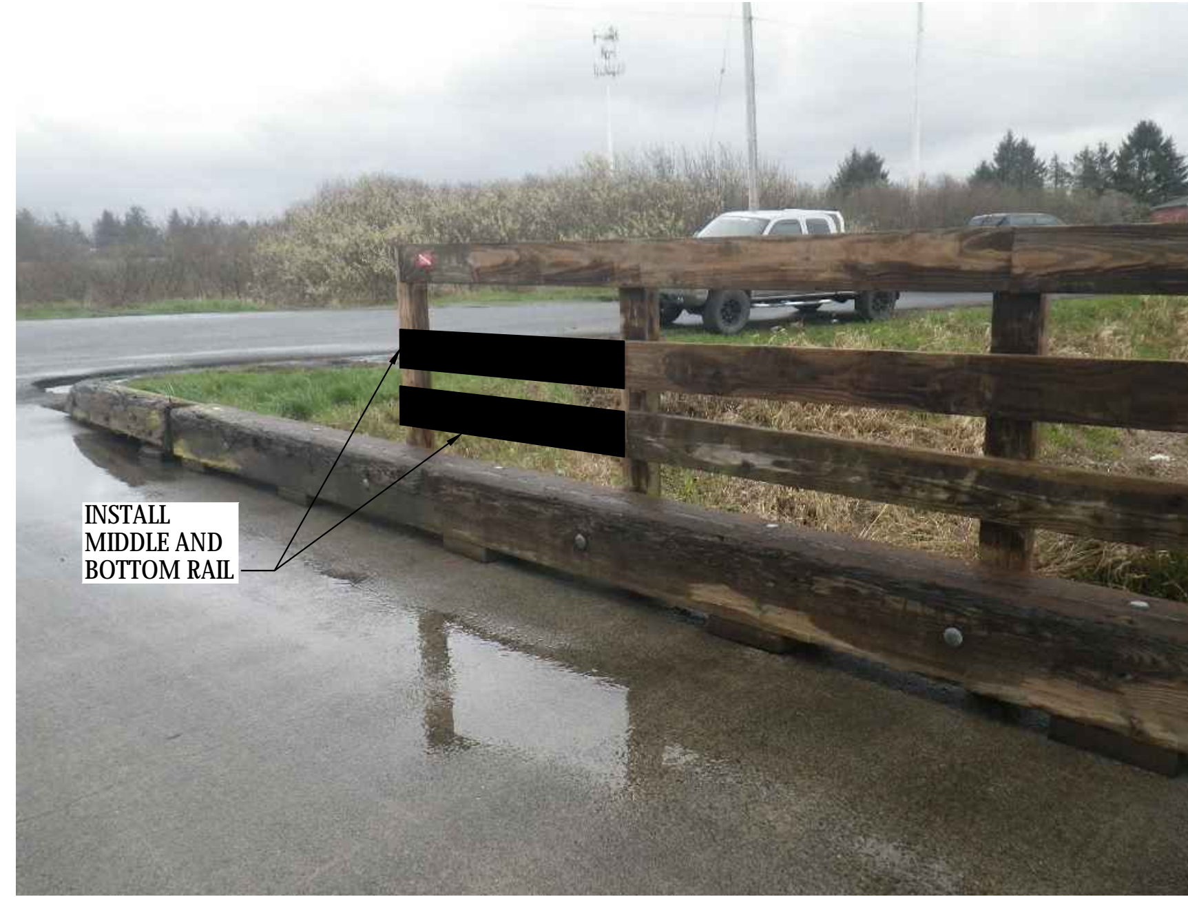
14 PHOTO - EAST TRESTLE RAILING 5-12 SCALE: NTS
