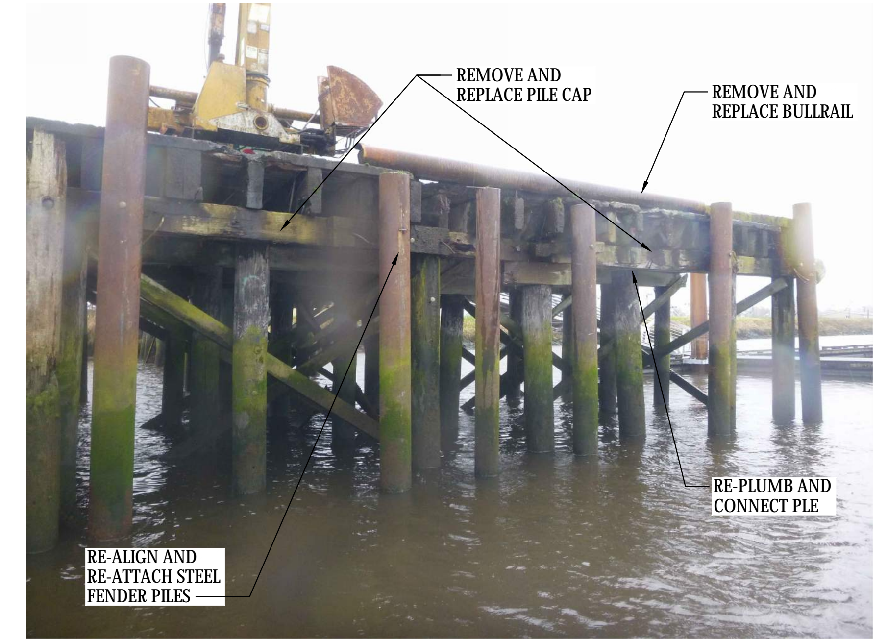
9 PHOTO - NORTH EDGE OF WEST TRESTLE S-06 SCALE: NTS
