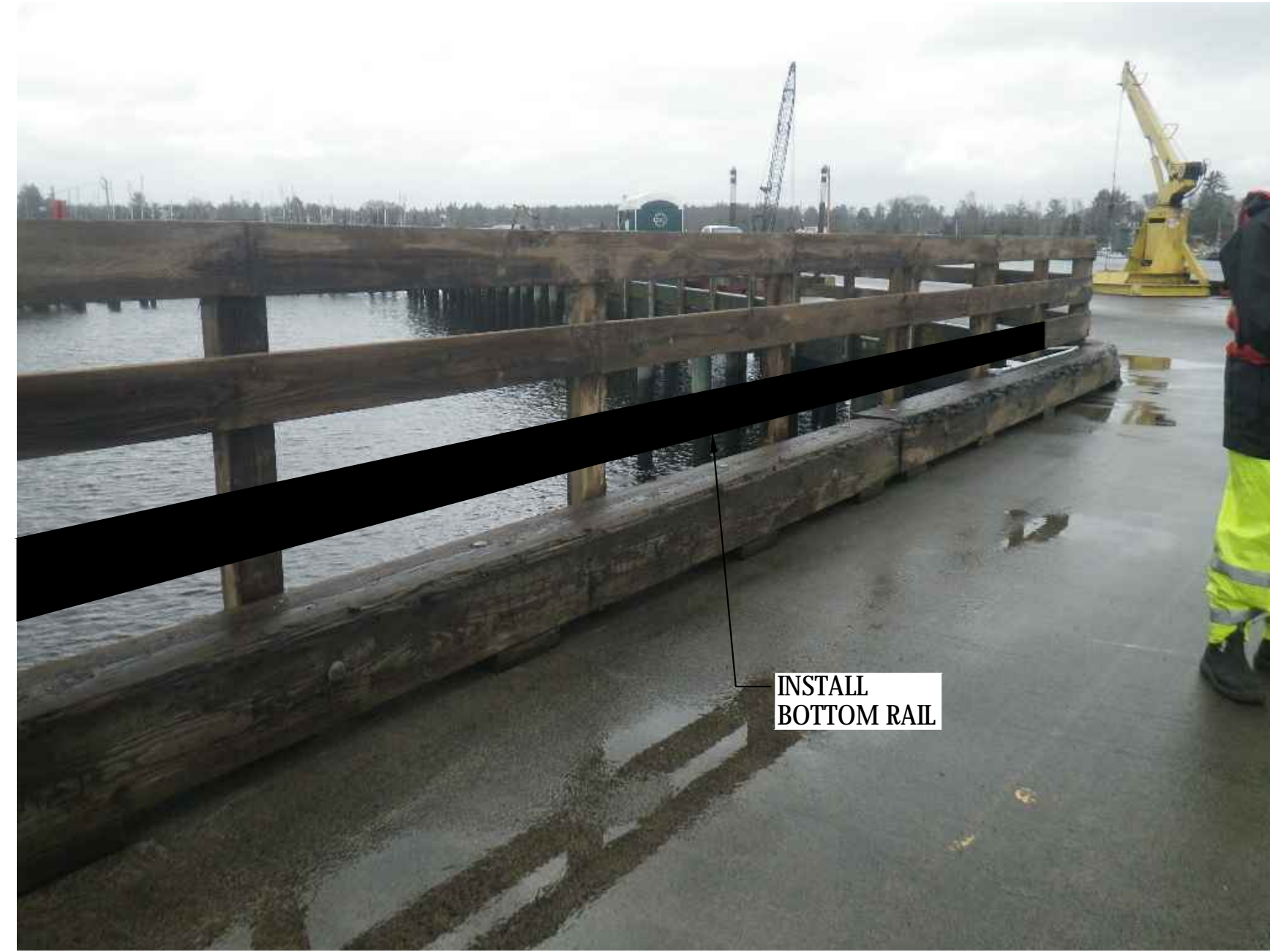
13 PHOTO - EAST TRESTLE RAILING 5-11 SCALE: NTS
